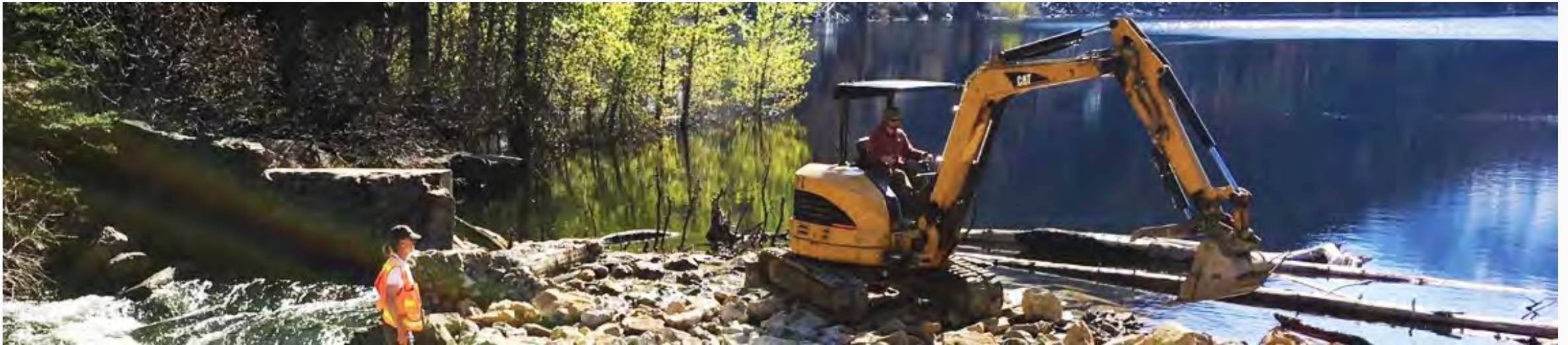
Emergency temporary construction at Eightmile Dam
